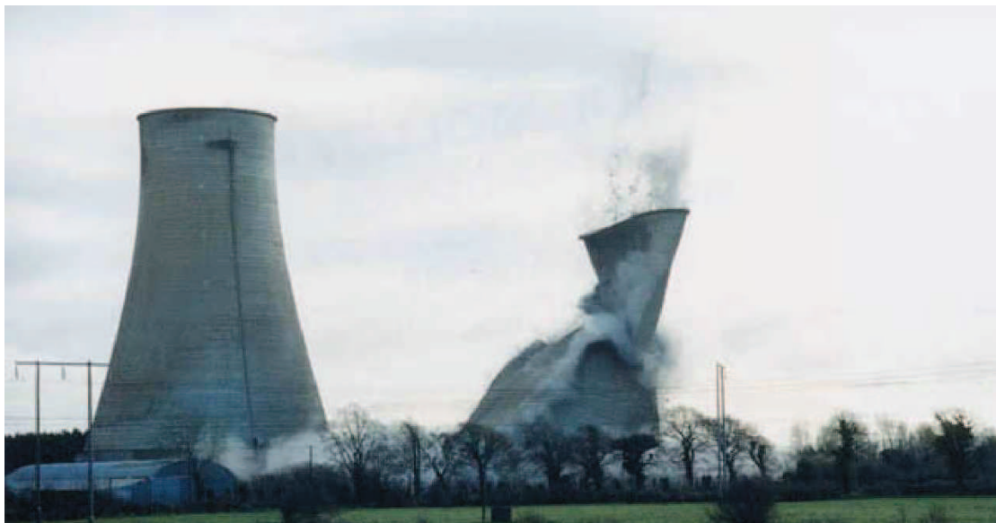
Figure 2.6 Demolition of the First Cooling Tower at the Former Ferbane Peat Fired Station
