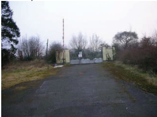
Existing site entrance – facing north
