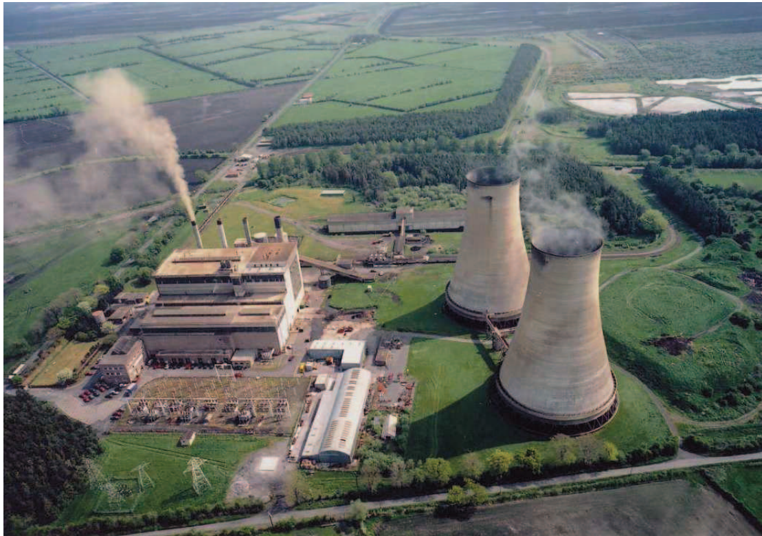
Figure 2.3 Aerial view of Former Ferbane Peat Fired Power Station
