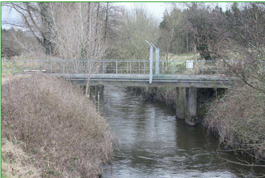
Figure 9.2.3 Local Access Railway access bridge ~32m upstream of Lumcloon Br.
