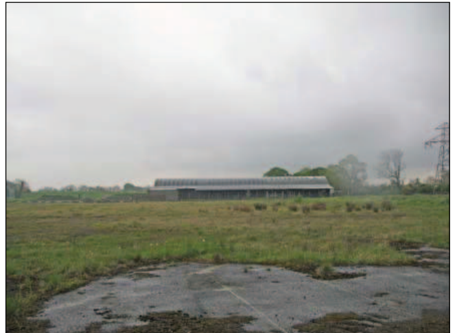
6.6.3 Application site looking south towards former site of cooling towers
