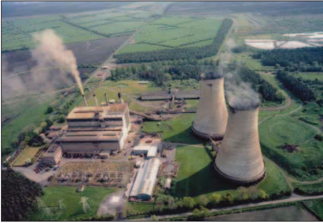
6.4.1 Historical oblique aerial view of former ESB plant
