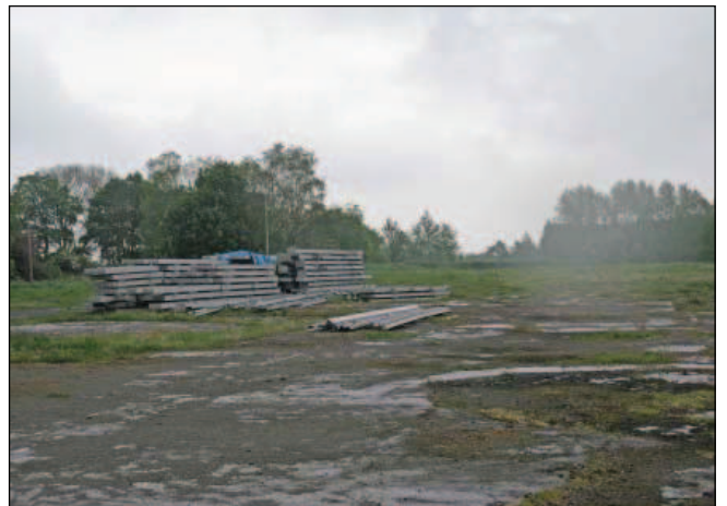
6.6.5 Storage of materials to centre of application site
