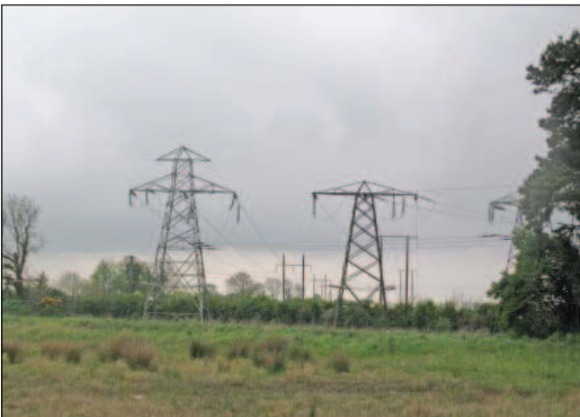
6.6.4 Existing pylons to west of application site
