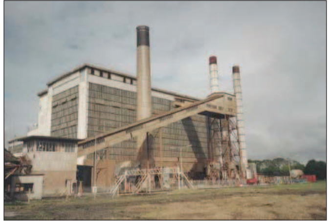
6.4.2 Former ESB plant (1990's)
