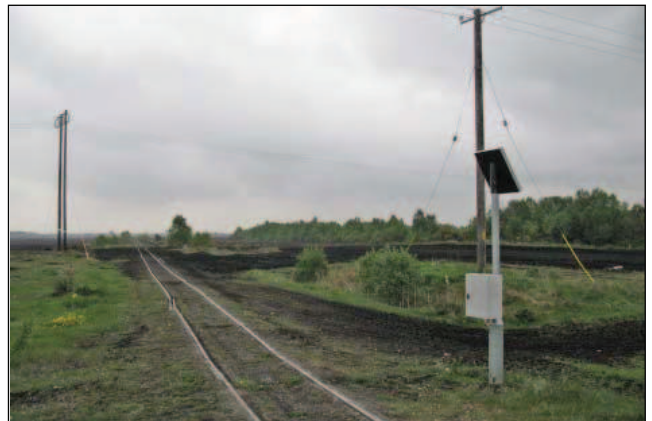
6.7.6 Industrial Rail across peatlands
